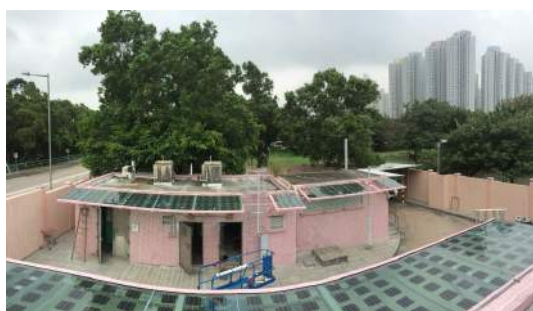
Pump station at Chung Mun Road, Tung Chung, Hong Kong Power output: 1.8kWp
